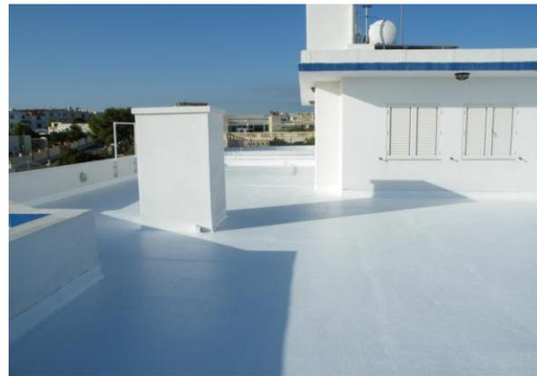
The glass fibre reinforcing further adds to the durability of the Acrylflex RRC.
